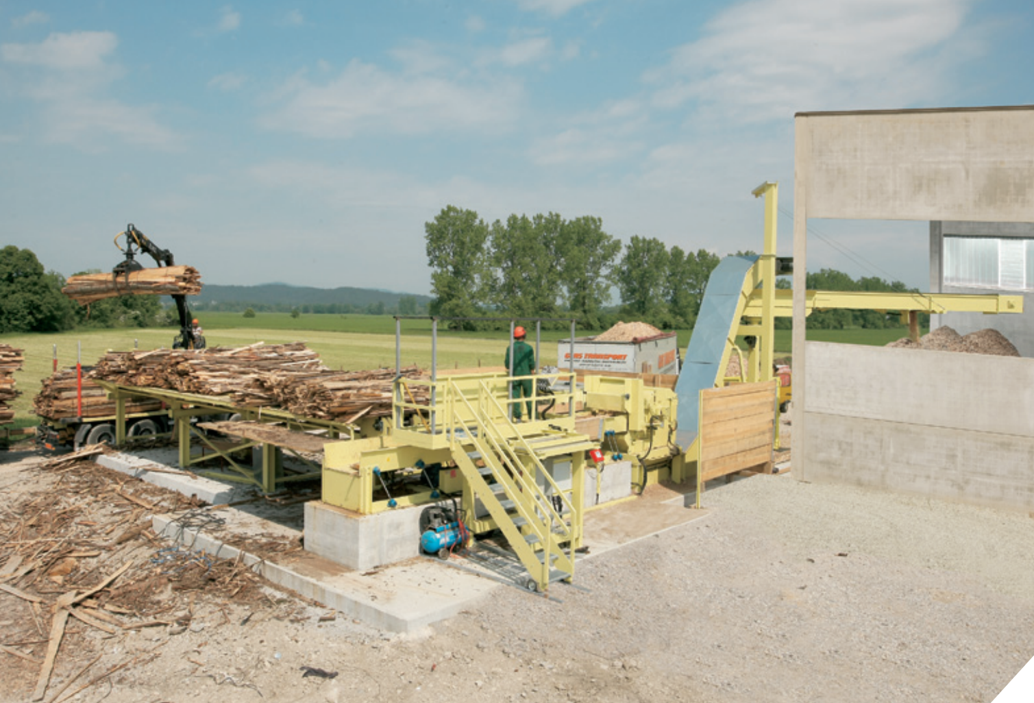
STATIONARY CHIPPING PLATS FOR SAWMILL TRIMS
